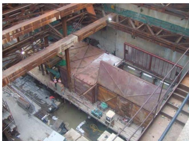
Noise enclosure provided at the launching shaft to contain localized environmental impact during TBM tunneling
